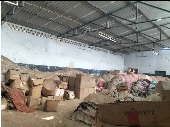
Internal View of Factory Shed.
