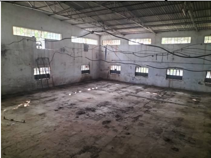
Internal View of Factory Shed.
