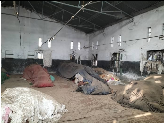
Internal View of Factory Shed.
