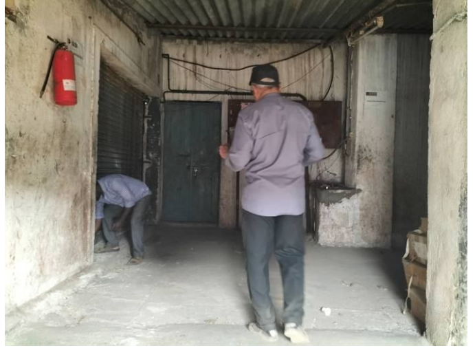
Internal View of Industrial Shed.
